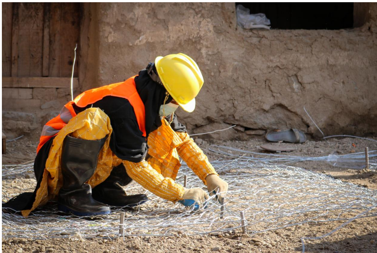
Figure 14: A returnee woman weaving gabion in a DRC supported project in Watapoor. Photo credit: Danish Refugee Council (DRC) Afghanistan.
